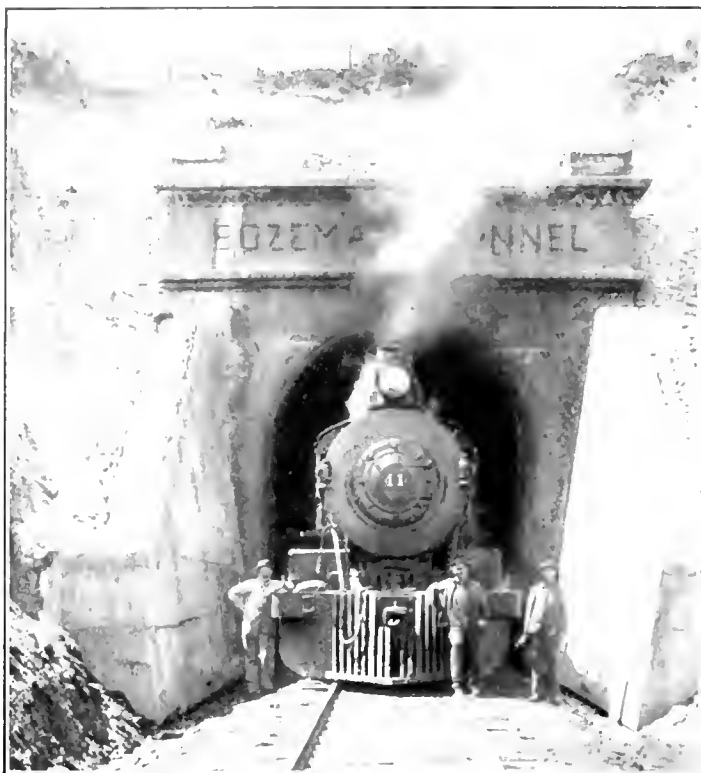
THE TUNNEL, SUCCESSOR TO THE SWITCHBACK Bored at a cost of a million a mile to save the high operating cost of the switchback. The Bozeman tunnel on the Northern Pacific
